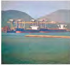
A view of the Gangavaram Port where an LNG terminal is to be set up. *K.R. DEEPAK
